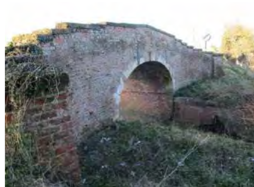
Photo 9: Strensall New Bridge
