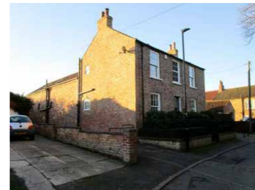
Photo 34: Example of detached house with rear wing
