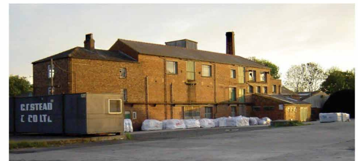
The Tannery, Strensall, now demolished
