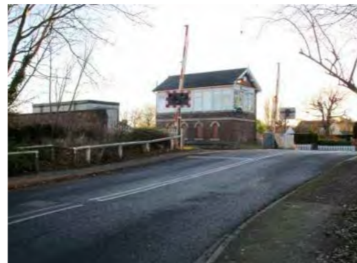
Photo 10: Level crossing at Lord's Moor Lane
