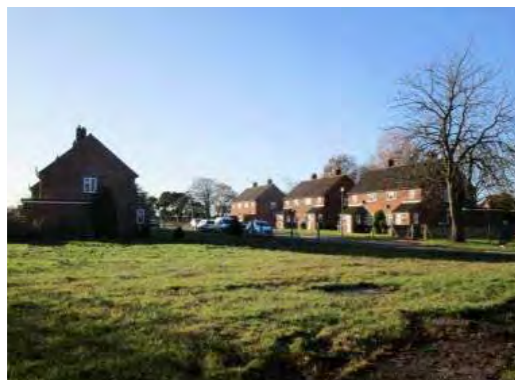
Photo 18: Housing along St Wilfred's Road
